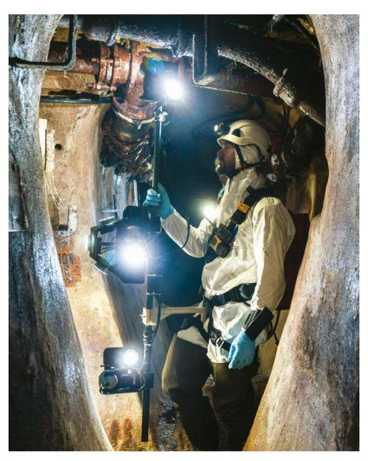
3D sewer mapping to facilitate management of a sanitation system (France)
